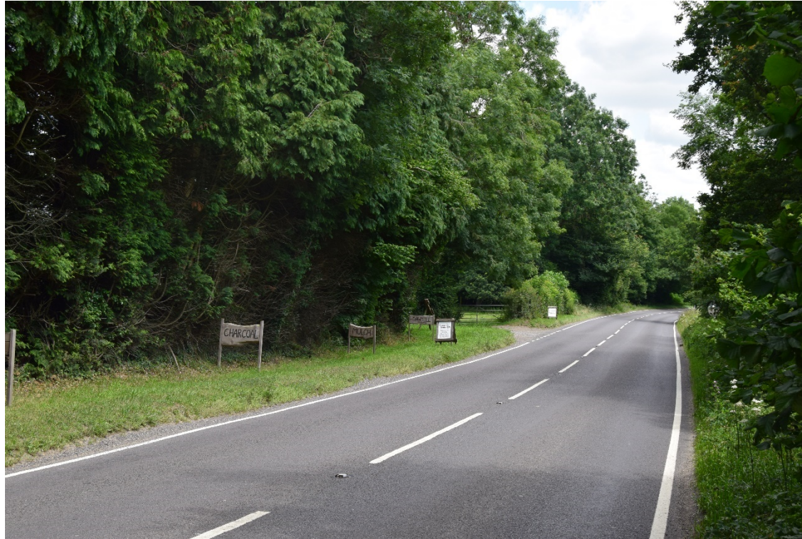
Figure BMFA.4 Site photograph 3 View east along A283 on northern boundary of SDNP showing previously proposed site entrance. Note: An alternative layout has since been proposed which proposes connecting this site to Rock Common Quarry in the west by a conveyor and thus negates the need for this access route.
