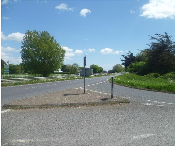
Photograph 5.1: Primary Direction Visibility Splay from Green Lane
