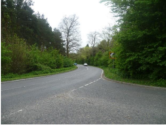
Photograph 11.1: The Hollow / A283 Primary direction visibility
