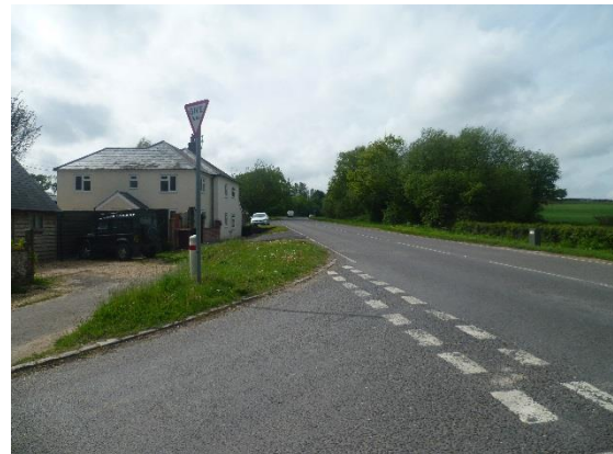
Photograph 6.2: Durford Lane / A272 secondary direction visibility splay
