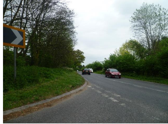
Photograph 11.2: The Hollow / A283 Secondary direction visibility
