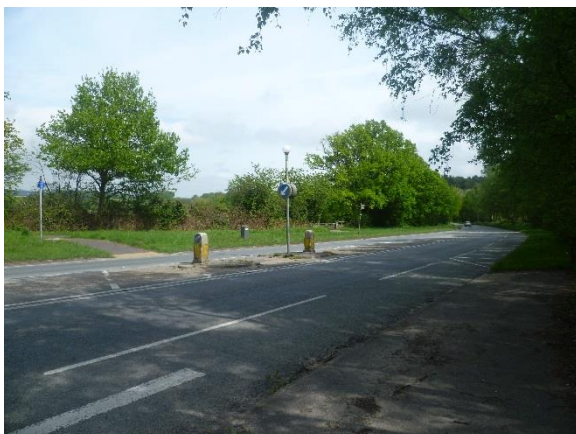
Photograph 7.1: Minsted Road / A272 view east
