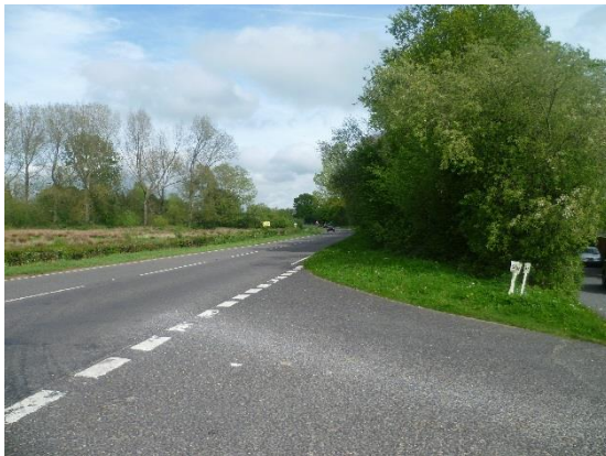
Photograph 6.1: Durford Lane / A272 primary direction visibility splay
