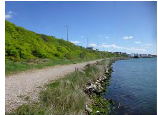
North Canal Bank
