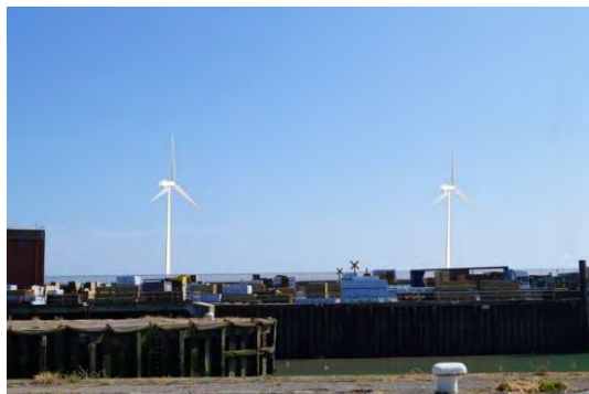
Wind turbines at Outer Layby
