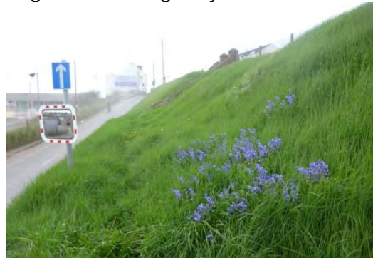
Basin Road North embankment
