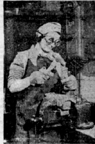
Mrs. Prodger, 18, Thackeray-road, Worthing, has been a factory worker in two wars. She works on white metalling and chipping of coach-bearing brass parts—much the same as she did in the last war. Her husband is in the Army.
