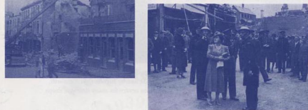
Below: The King and Queen inspect flying bomb damage, East Grinstead, July 1944
