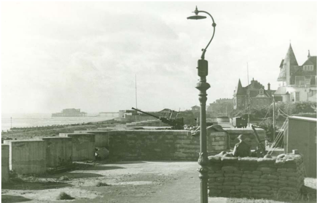
Gun emplacement at Splash Point, Worthing (PP/WSL/WGP000025) www.westsussexpast.org.uk/pictures
