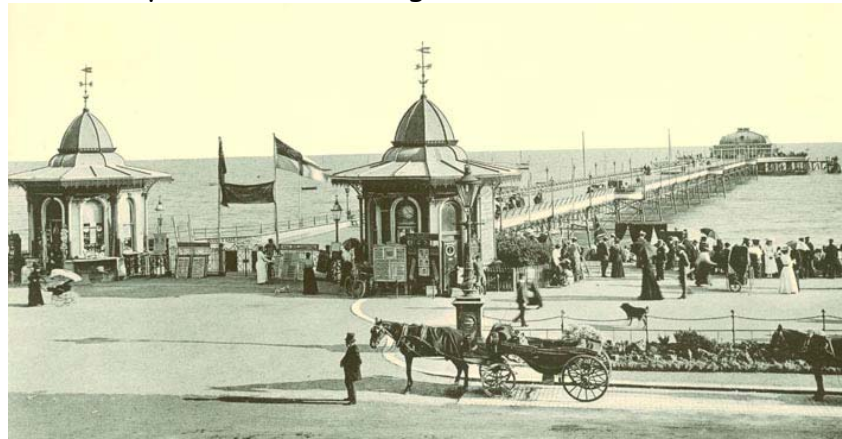
36f. The pier c1889, looking south east
