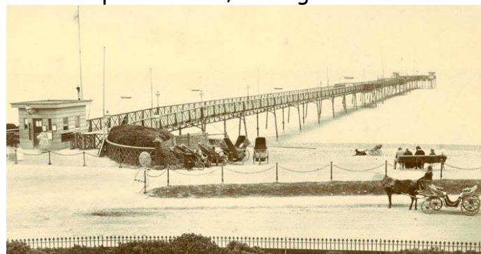
36d. The pier in 1886, looking south east
