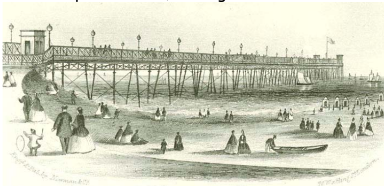
36b. The pier in 1866, looking east
