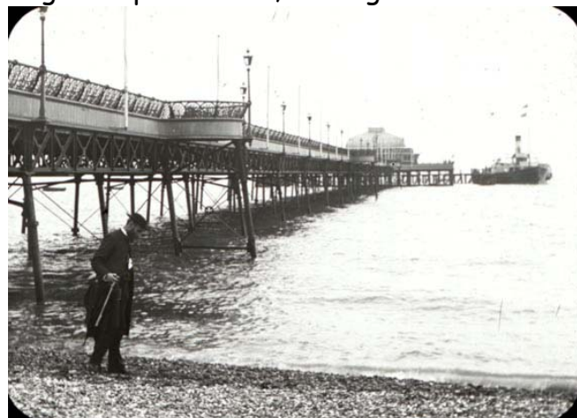
36g. The pier c1900, looking south east
