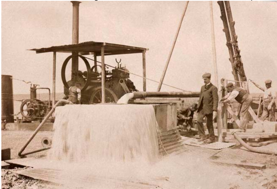
Source 2. D&O workers testing water flow from a borehole, Littlehampton, c1900
