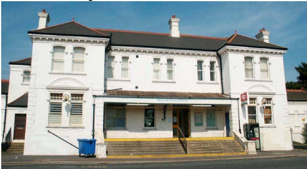
The south side of the station building
