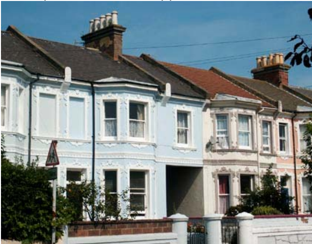
Houses on the north side of the road.
