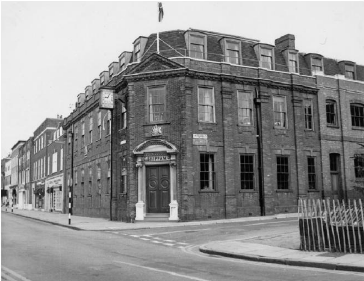
Former factory of Shippam's in East Street, Chichester West Sussex Record Office, Shippams collection
