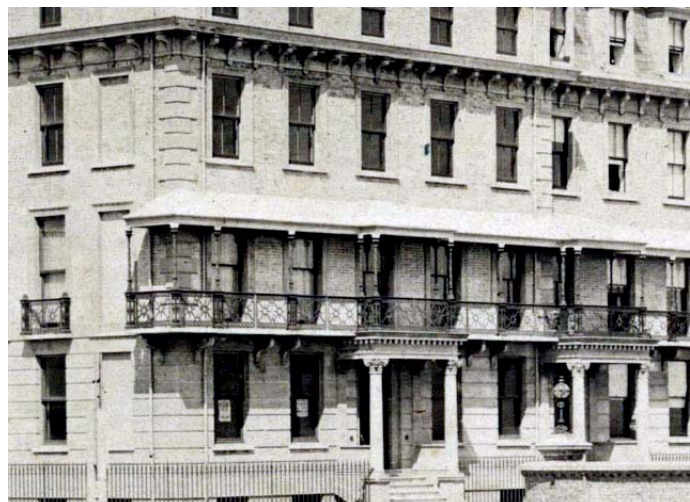
A close view of the south west corner.
