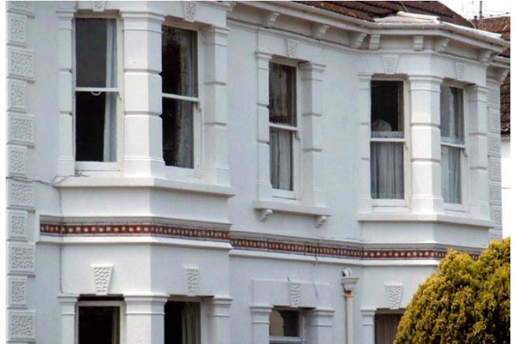
A close view of the house on the right,
