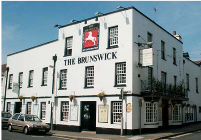
The south and east sides.
