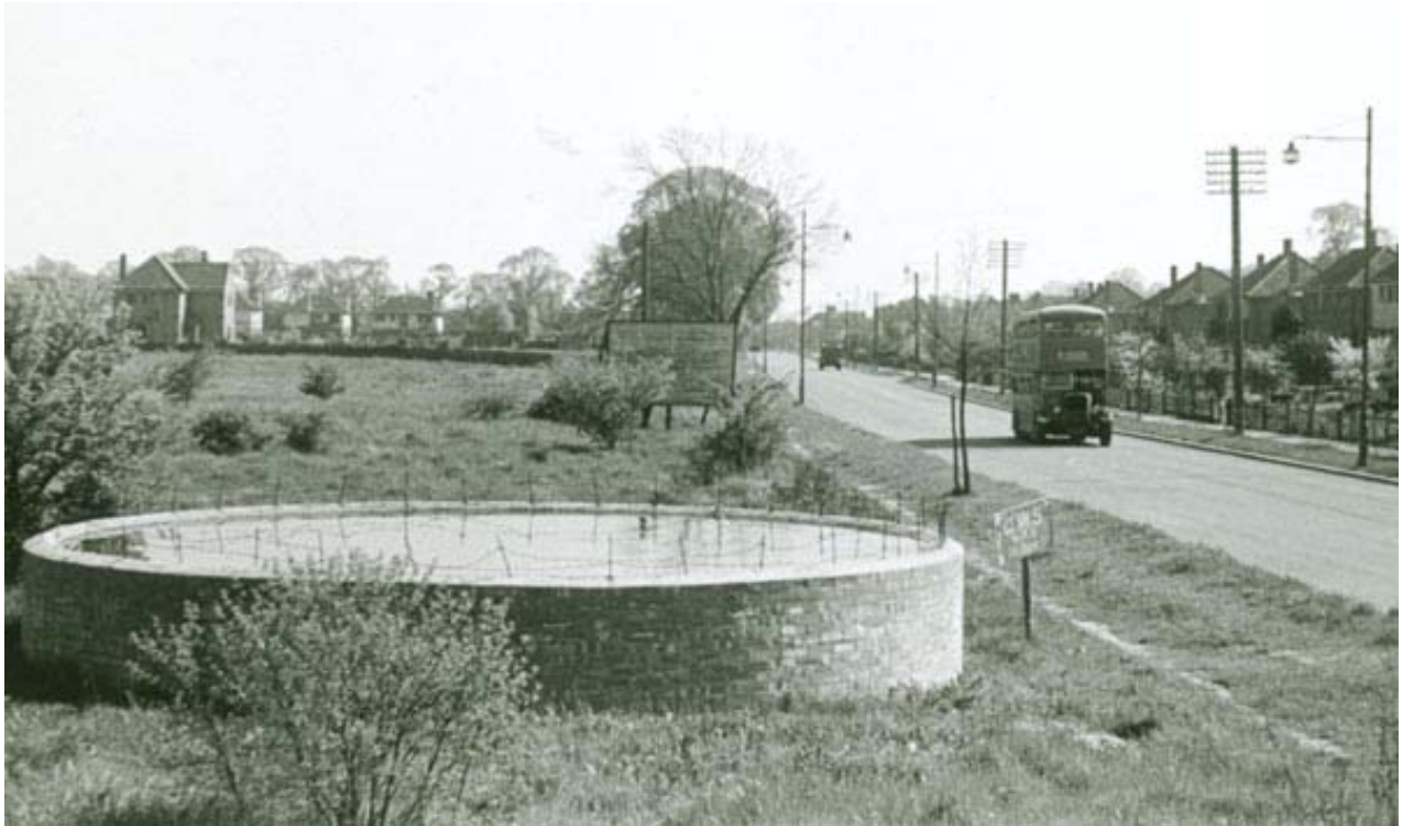
Emergency water supply tank on Findon Road
