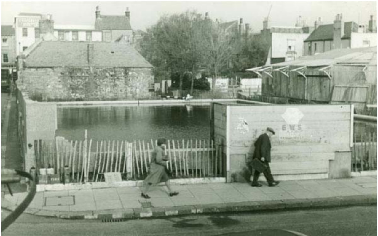
Emergency water supply tank in Worthing
