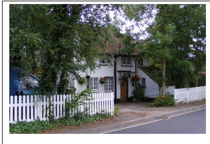
4 St Leonards Road 'Well Cottage' – 2010 Authors photo.
