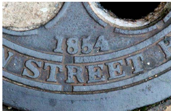
35b. Close detail of Heene Terrace coal hole cover
