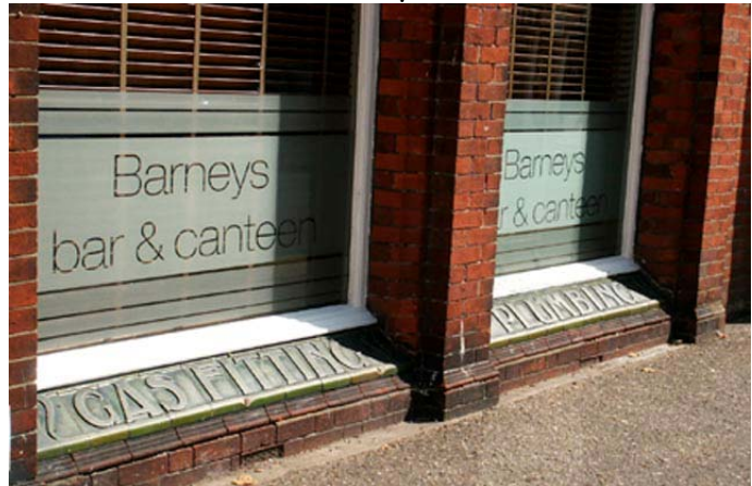
Close view of part of the west side of the building.
