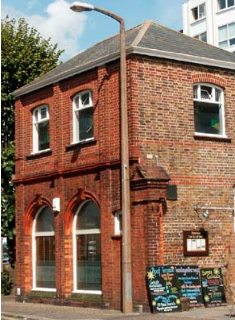
West and south sides of the building.
