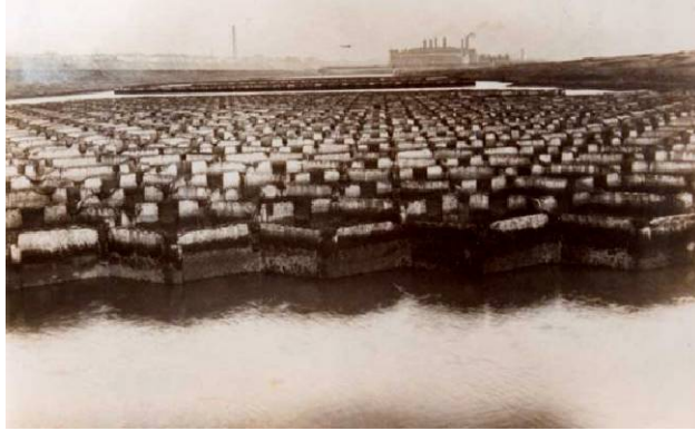
Bases of unused Mystery Towers at Shoreham Harbour in 1930. The honeycombed structure can be clearly seen. These unused bases became the foundations for the Southwick Power Station in 1947. Courtesy of West Sussex Record Office reference number Photographs/PH/16959
