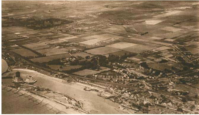
Aerial photograph of Shoreham Harbour circa 1919. The Mystery Towers can be seen in the lower left corner and the workers hutted encampment is on the right. The Slonk Hill army camp is at the top-centre. Courtesy of Marlipins Museum reference number PP/SHORM/93.2220 ( www.westsussexpast.org.uk )
