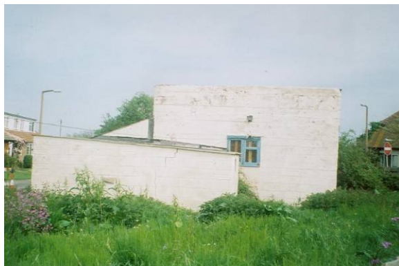
The Selsey Sound Mirror in 2008. The window that has been cut through the curved face can be seen. Courtesy of Andrew Grantham www.andrewgrantham.co.uk
