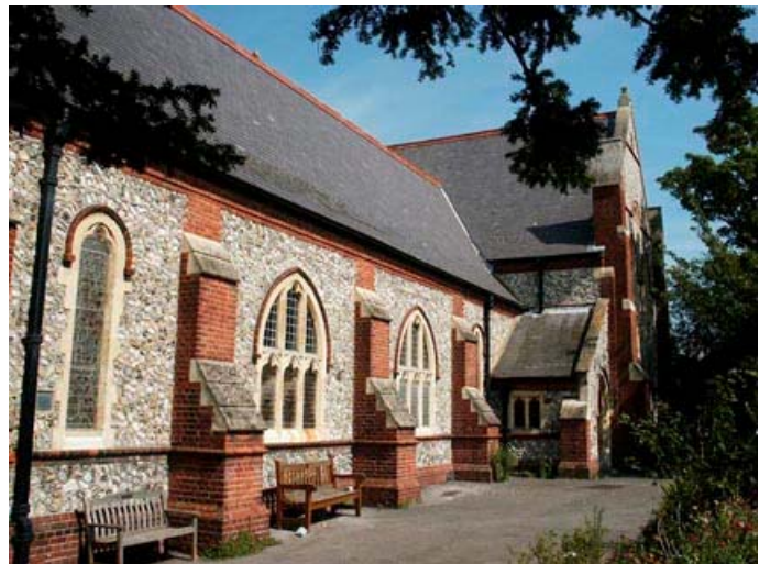
The south side of the church on Manor Road.
