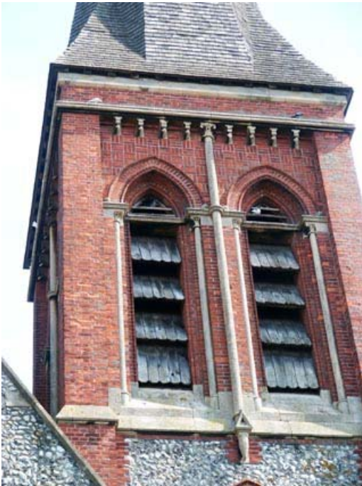
Close view of a detail of the steeple.
