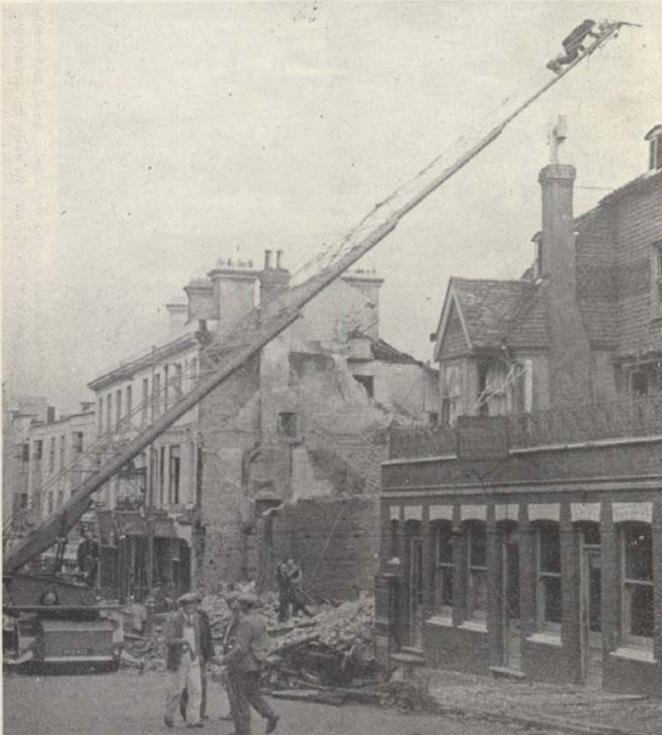
Fire fighting in London Road after the tragic raid on East Grinstead on July 9th, 1943
