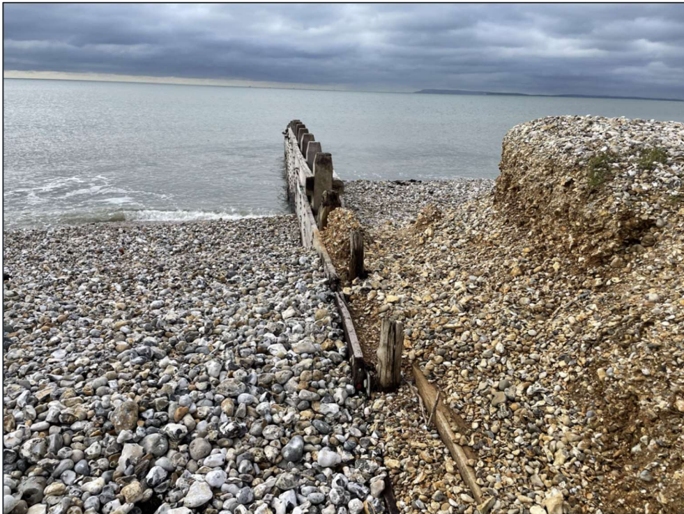
Figure 5-5 - Environment Agency's Sea Defence at Medmerry (taken 02/10/2024 - note drop in crest level)
