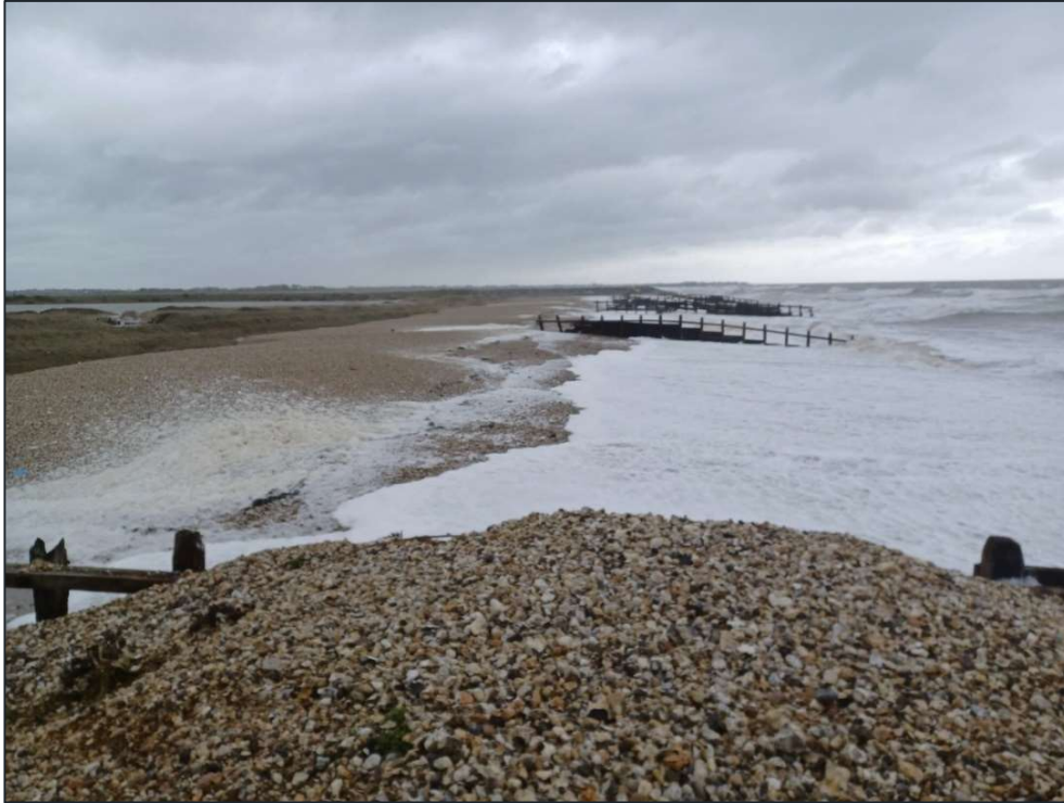
Figure 5-5 - Environment Agency's Sea Defence at Medmerry (taken 02/10/2024 - note drop in crest level)
