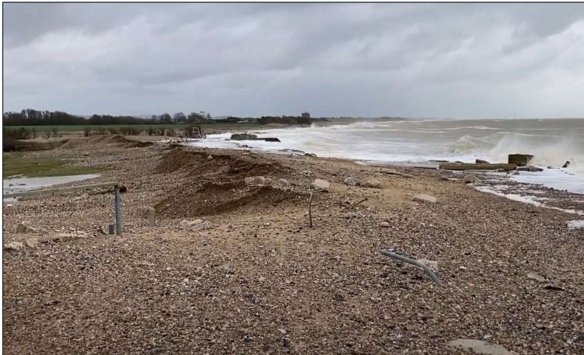
Figure 5-1 - Eroded Coastal Defences at Climping Beach (taken 9th April 2024)
