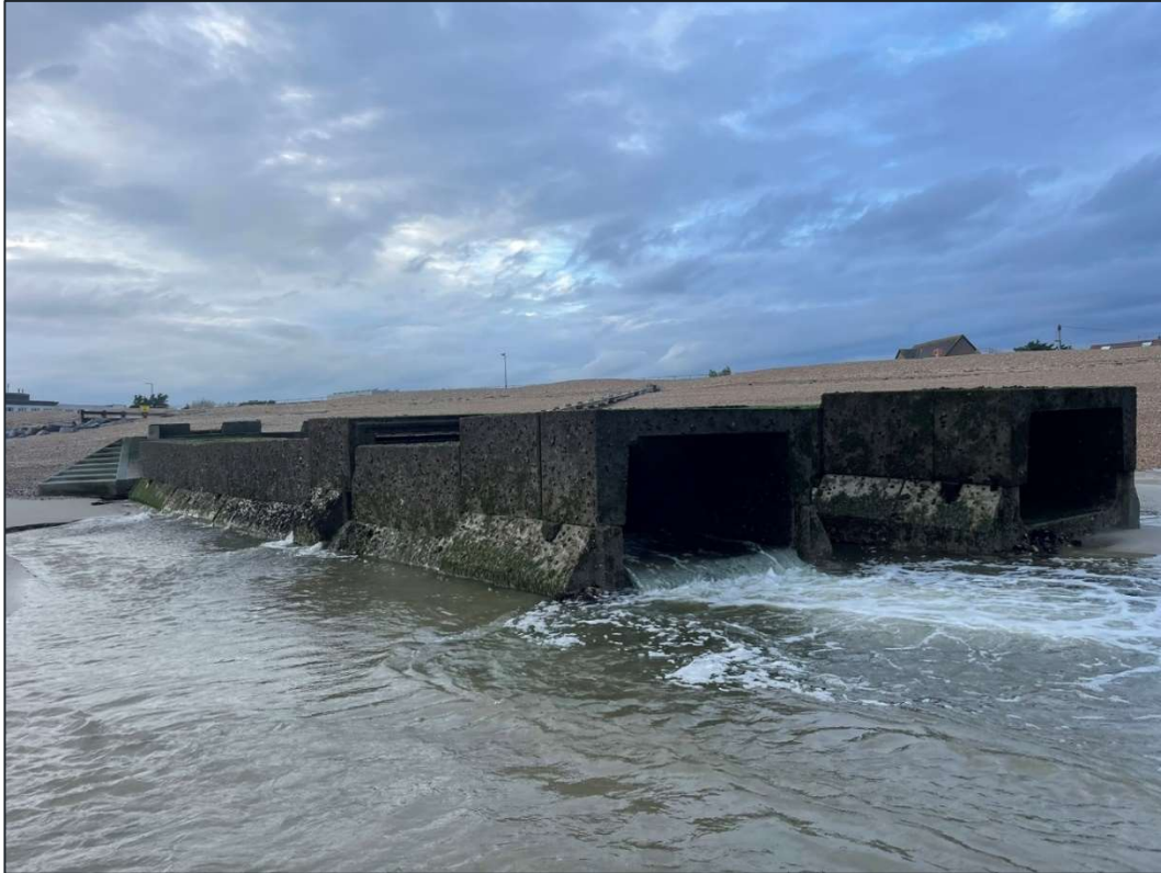
Figure 5-6 - Aldingbourne Rife Sea Outfall (note displaced culvert sections) (16/10/2024)
