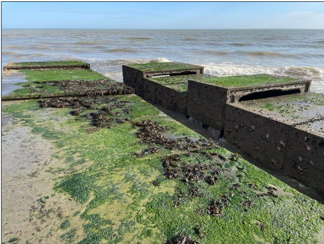
Figure 5-6 - Aldingbourne Rife Sea Outfall (note displaced culvert sections) (16/10/2024)
