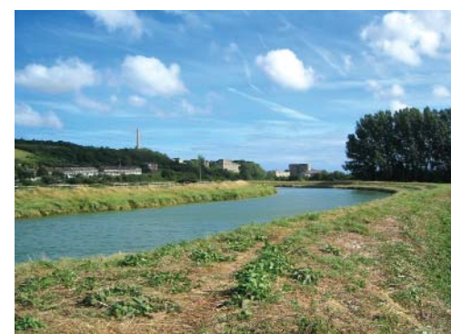
Views across the tidal River Adur to Shoreham cement works
