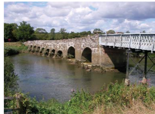
Greatham Bridge - stone
